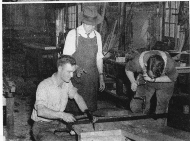
Lacy Smith straightens the axel of a truck while John Rochon holds it securely in place on the anvil. Much work of this type is done on the forge in this branch of the Carpenter Shop.
